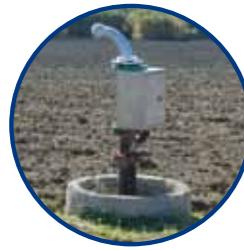
DARA UPDATING ( WATER CONSUMPTIONS AND CONFIGURATION) FROM FIELD DEVICES VIA GPRS
